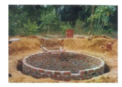
Figure 10: Outlet of the tank
