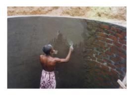
Figure 12: Plastering the tank
