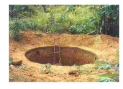
Figure 3: Pit for the tank construction
