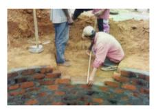
Figure 6: Measurement taken for the inlet construction
